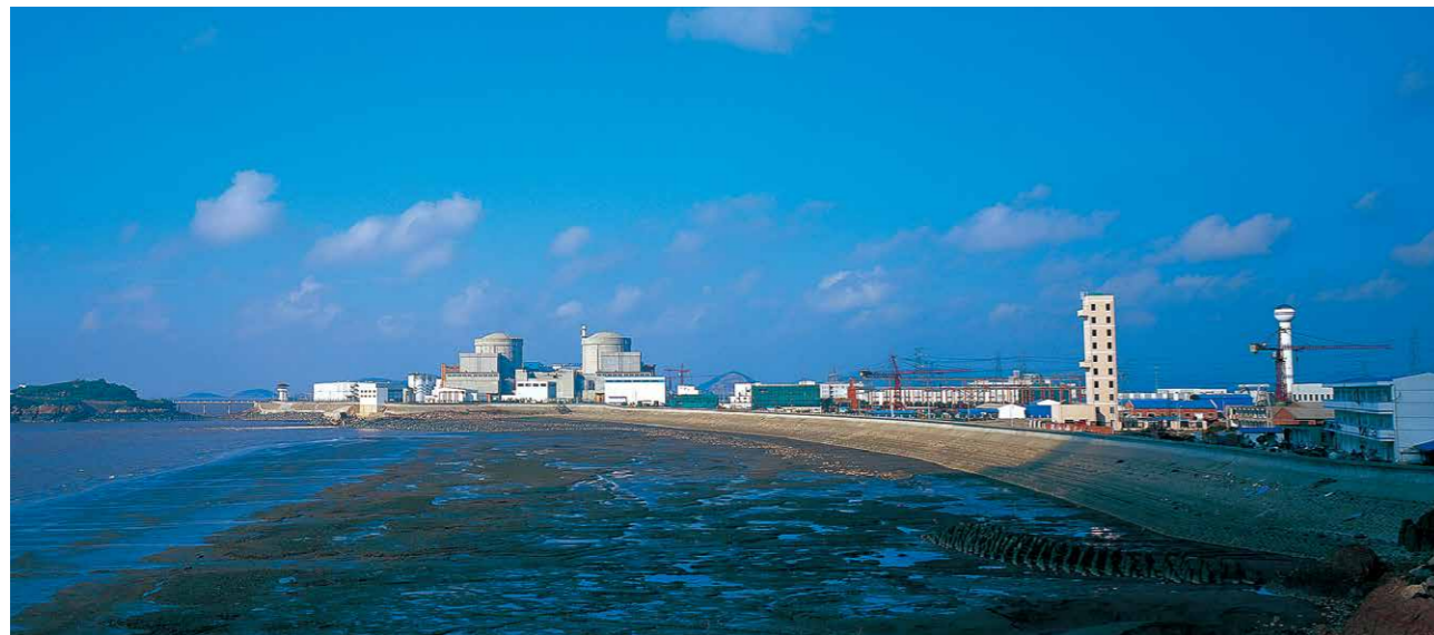
Qinshan Nuclear Power Plant Phase II Project Units 1 and 2
