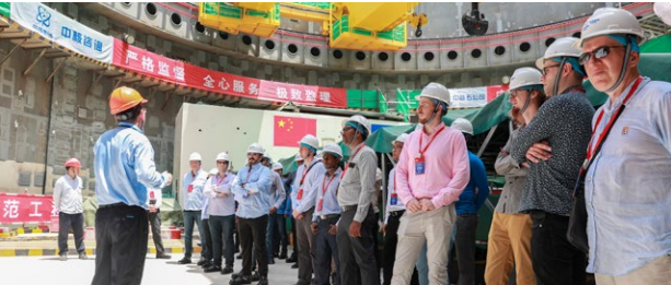
The visit to the small modular reactor construction site
