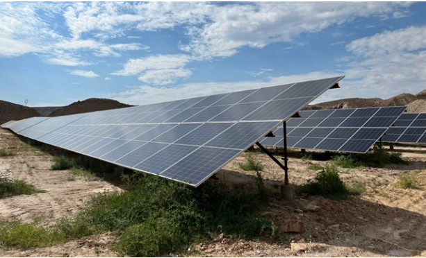
Copper and mine waste quarry tailings treatment photovoltaic project in Baiyin, Gansu Province- Post-treatment geomorphic vegetation
