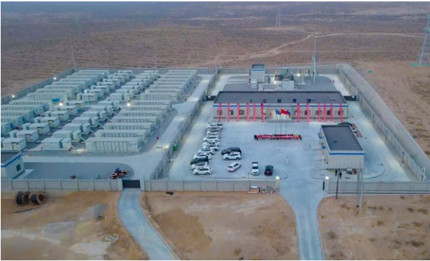
CNNP Rich Energy Co., Ltd. constructed a energy storage power station in Tongxin County
