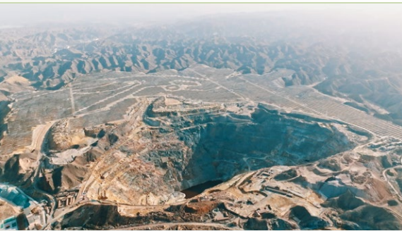
Panorama of the solar PV project to treat tailings in the waste rock field of the Baiyin deep copper mine
