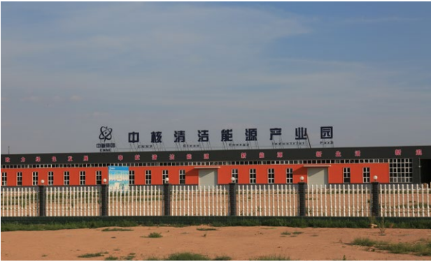
Clean energy industrial park of CNNP Rich Energy Co., Ltd.
