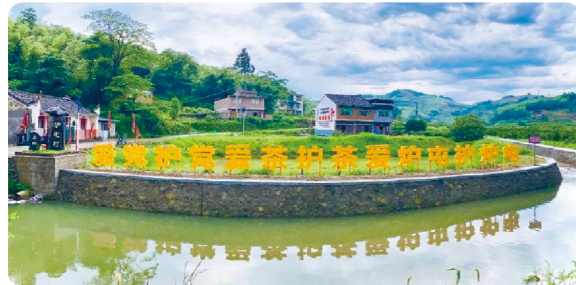
The riverbank in Lutun Village built with the support of Fuqing Nuclear Power Plant
