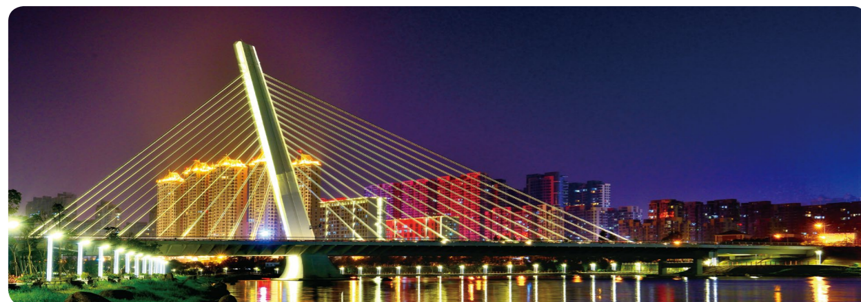
Guanyinpu bridge in Fuqing city co-built by Fuqing Nuclear Power Plant and the local area
