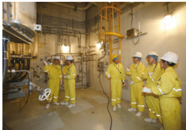
PSUR for Sanmen Nuclear Power's No.1 unit
