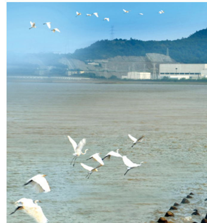
Egrets Flying over the Nuclear Power Plant
